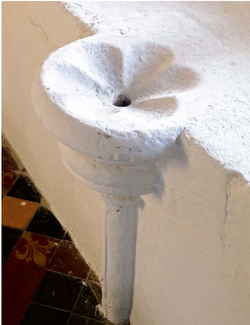
Piscina in All Saints Church of England, North Moreton, Oxfordshire. Dating from ca. 1270, the piscina's unusual cinquofoiled basin forms the capital of a small shaft containing the drain. Courtesy John Ward.
